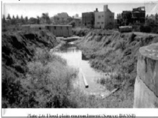
Plate 2.6: Flood plain encroachment (Source: BBWSII) Fig No: 7 Encroached Drainages in Bangalore BBMP
