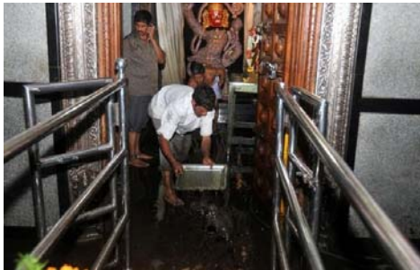
Fig no: 11 Ghali Anjaneya temple flooded on Nov 9 th -2014
